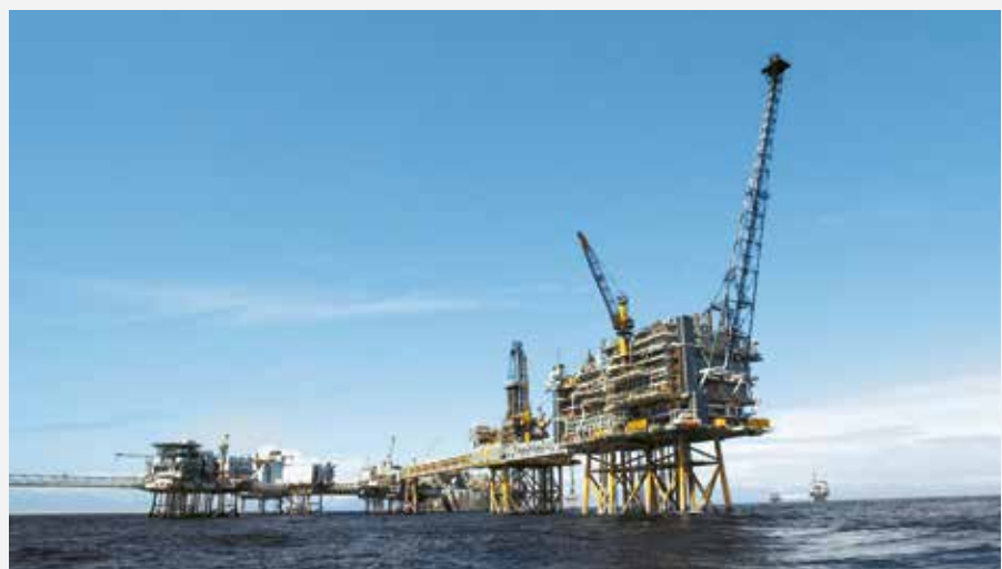
Industrial gas turbines ensure that oil rigs are energy self-sufficient.
