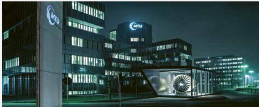
MTU Aero Engines' headquarters and – with over 4,700 employees – largest production site is in Munich. A traditional aviation site, Munich is inextricably linked to the history of powered flight – its roots reaching back to the early 20th century.
