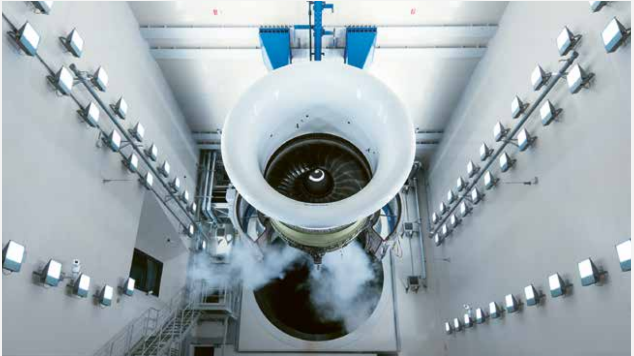
A freshly overhauled GE90 Growth engine must undergo an acceptance test run—in line with the scope of the shop visit. There are two test cells at the Hannover location: with a thrust range up to 100,000 pounds and 150,000 pounds, respectively.
